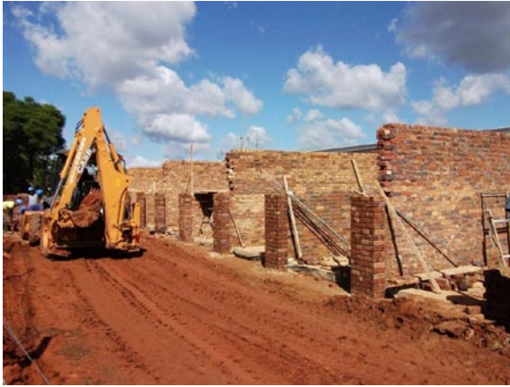
Ground floor brickwork to block F nearing completion
