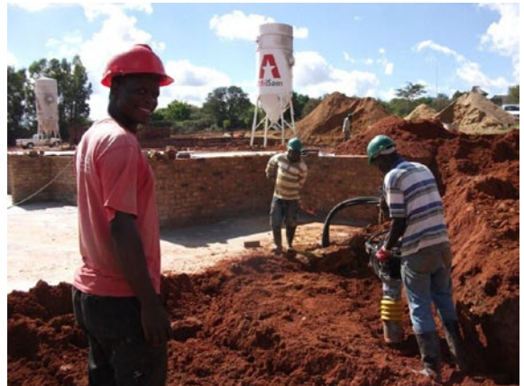
Compaction to road underway
