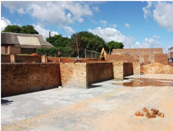
Retaining wall to block G substantially complete
