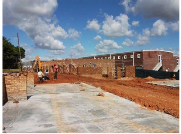
Floor slab for block G complete
