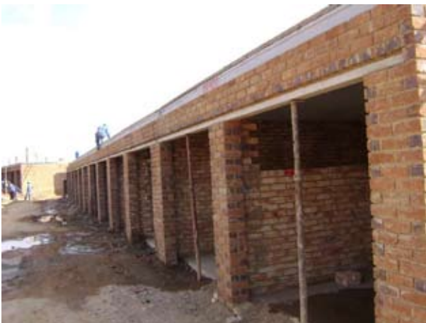
First floor slab to Block C complete
