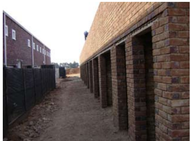
First floor brickwork to Block F nearing completion
