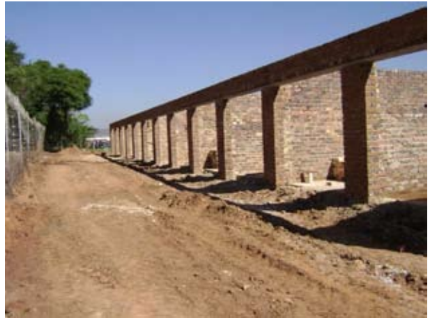
Ground floor brickwork to Block C complete
