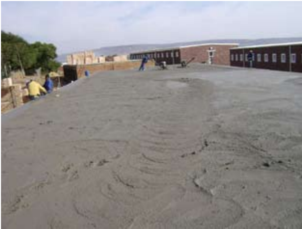
Power floating to Block F first floor slab underway
